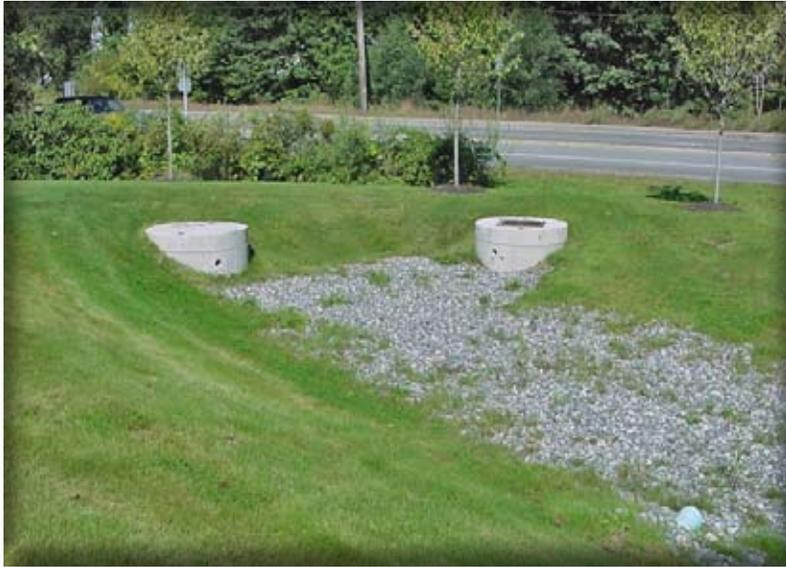
**Description:** Infiltration basins are stormwater runoff impoundments that are constructed over permeable soils. Pretreatment is critical for effective performance of infiltration basins. Runoff from the design storm is stored until it exfiltrates through the soil of the basin floor.
